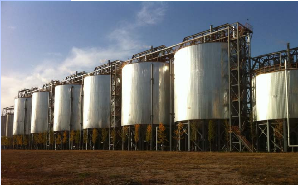
Red mud decanter and washer circuit using deep cone type thickeners
